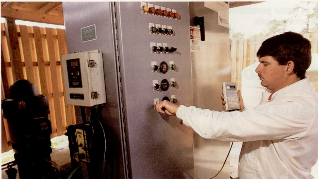
When Gator Creek Superintendent Mark Todd checks his VFD pump system, he reads the digital screen on his operator interface device (OID) and easily scrolls through complete diagnostic and historical information stored in the system.
