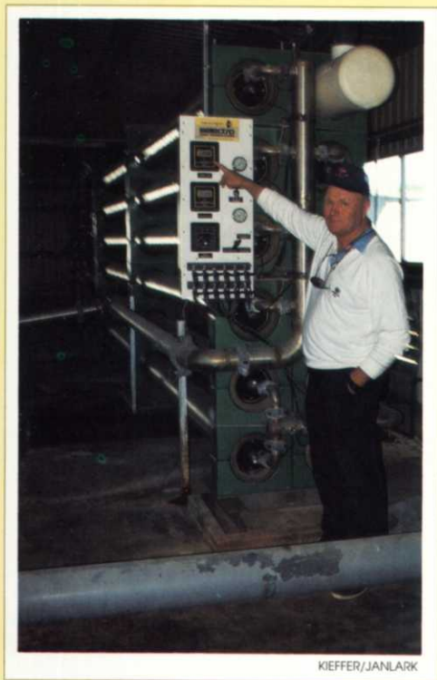
Ray Hansen at the controls of one of the reverse osmosis units.
