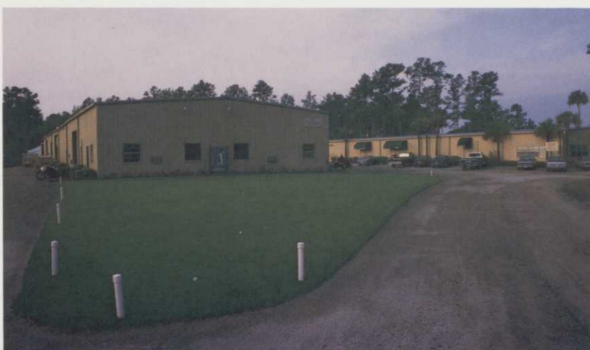
TPC Maintenance Complex
