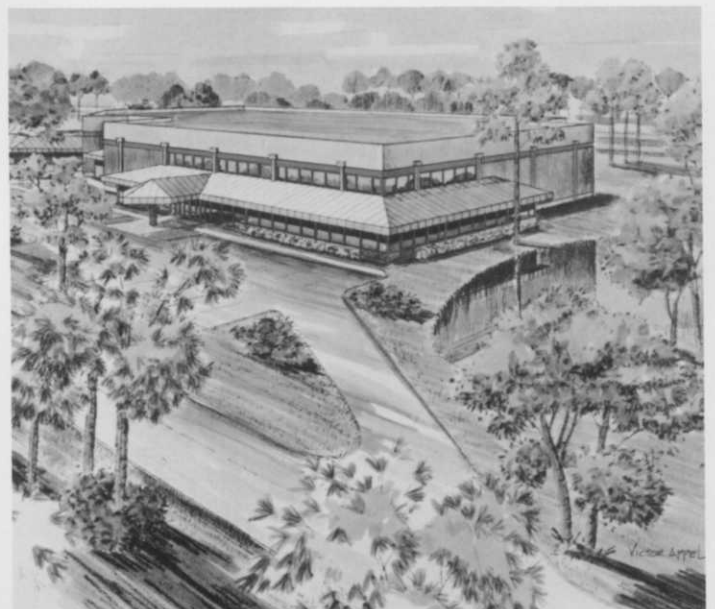
Wesco-Zaun's new distribution facility.
