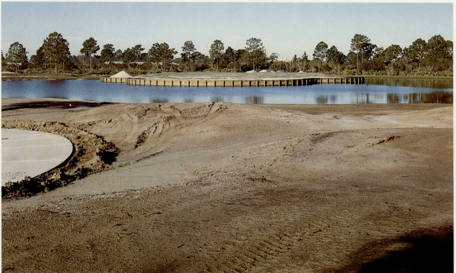
The new Panther Golf Course under construction at Plantation.
