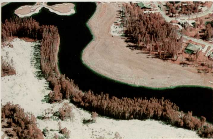
The two dark spots, immediately forward and to the left of the tee at Fiddlesticks in Ft. Myers, are subsurface leaks in the irrigation line. Not detectable from the surface.
