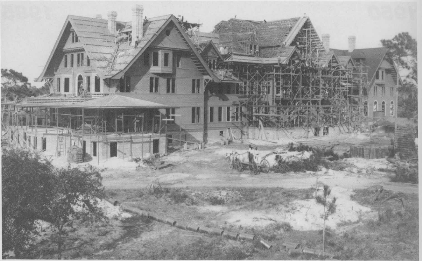
Construction of Biltmore Hotel in 1895-1896.
