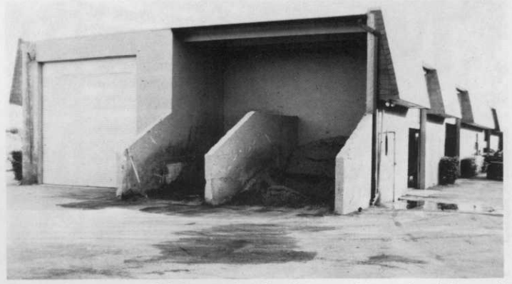
Boca Greens soil bins individually partitioned with roof overhand and high rising garage doors for easy entry.
