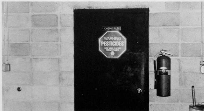
Highridge C.C. exemplifies properly locked metal chemical room door with signs posted and fire extinguisher.
