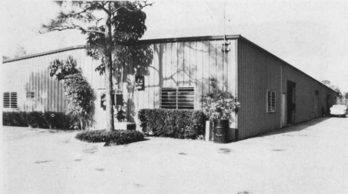
Frenchman's Creek maintenance building is perhaps one of the largest covered buildings in the country.
