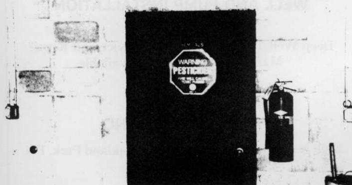
Highridge C.C. exemplifies properly locked metal chemical room door with signs posted and fire extinguisher.
