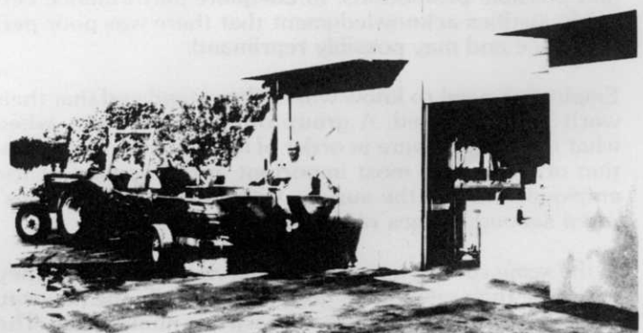
Boca Greens chemical room is designed with easy entry, concave floor with drain, sink, and outside hose bib. ■
