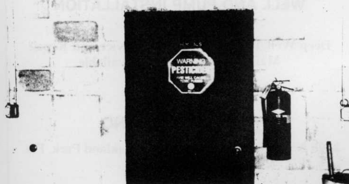
Highridge C.C. exemplifies properly locked metal chemical room door with signs posted and fire extinguisher.
