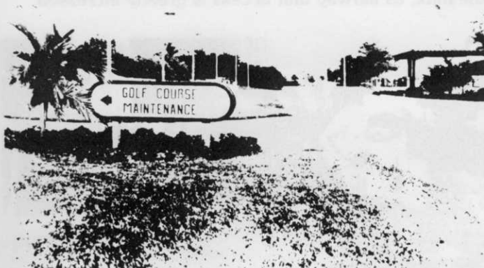
It is ideal for maintenance building to be well marked for easy delivery access along with proper landscaping.
