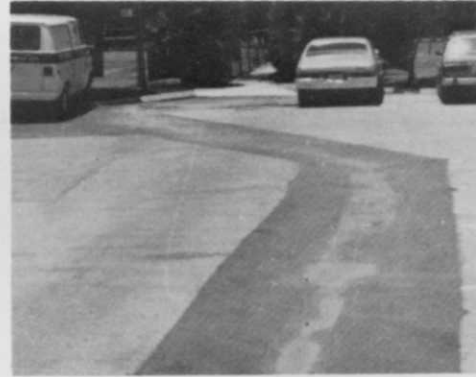
1. Brad Kocher and Rick Hammond are shown with inexpensive "Catch Basins" their crew made from concrete pipe "culls." In picture 2, we see Brad inspecting drainage ditches dug by his workmen. Even the paved parking lots collect water . . . in picture 3, you can see drainage swales installed by Inverrary's crew. Picture 4, is "mosquito control rig" made by Brad's mechanics. These shots show graphically that our members do more than GROW GRASS!
