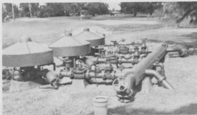
At Coral Ridge the problem was low water pressure as 3 turbine pumps drew water from small lake. Inefficient system had evolved from many add-ons over the past years. In picture 5, you can see the workmen starting to "untangle" the pipes. In picture 6, you see the 14" "header-pipe" being tailor-made to couple the pumps. In picture 7, you can see the finished product looking much better and working great!
