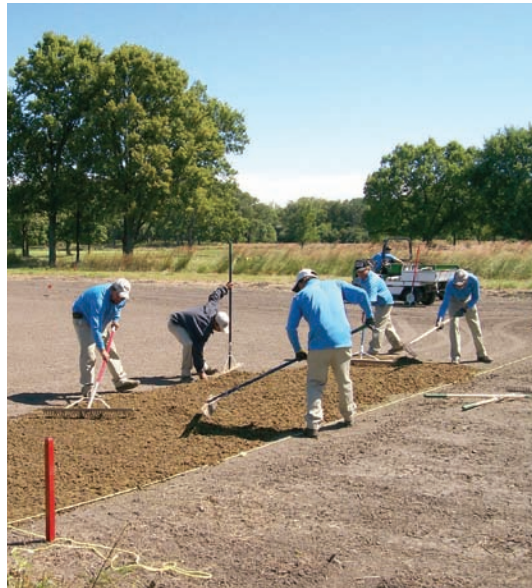
The cores are then spread out by hand on the prepped site to a depth of 1" or so.
