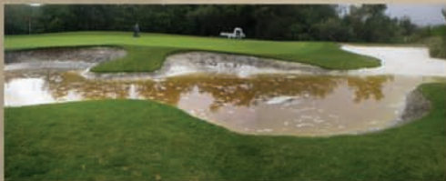
Before: Flooded Sand Trap
