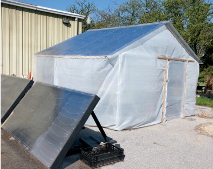
Briar Ridge's newly constructed greenhouse uses water heated by solar collectors to keep things on schedule for a spring planting.
