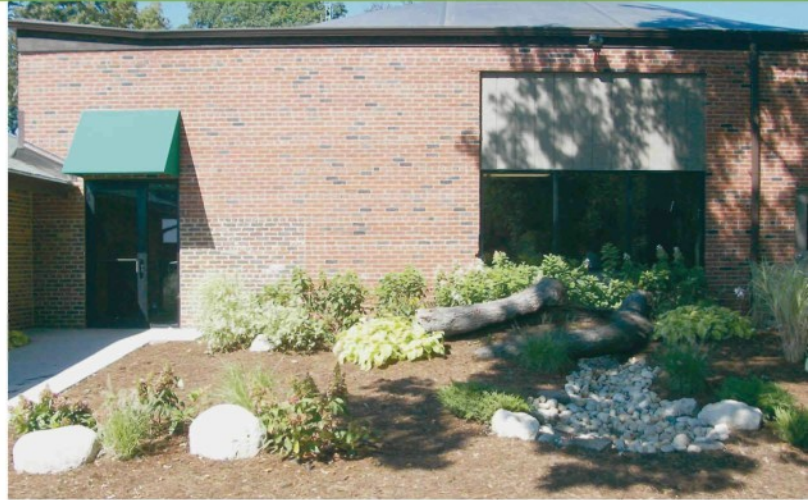
The new front entrance of Medinah Country Club's Turf Care Facility.
