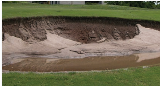
High flashed sand faced bunkers are nice to look at, but ding the labor line every time downpours hit.
