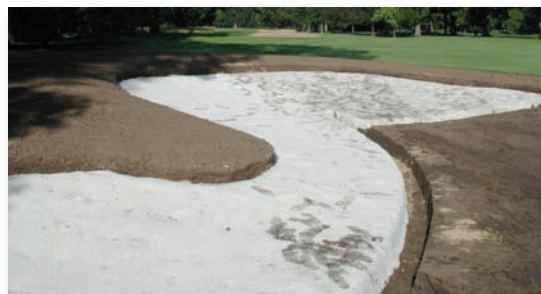
Bunker fabrics help to reduce labor and reduce sand contamination.
