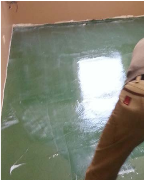
Dan added a coat of concrete semi-gloss to the floor to keep it shiny and easy to clean.
