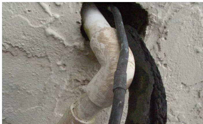
A lot of energy is lost where pipes run through exterior walls. Cans of expanding foam are a simple, inexpensive fix.
