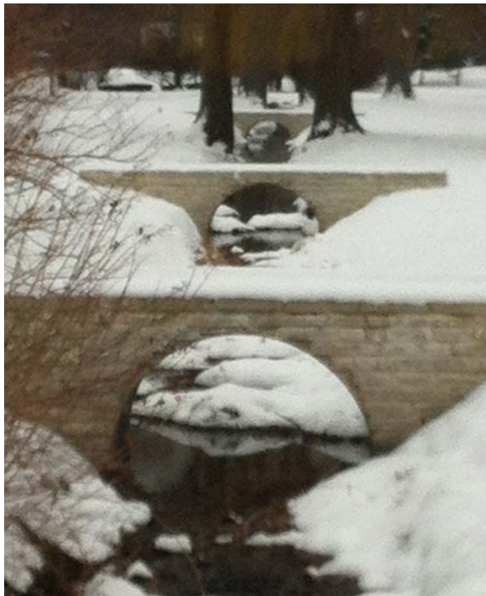
After the pipe was set in the ditch and footers were poured, skilled staff members at Indian Hill Club began the stonework.
