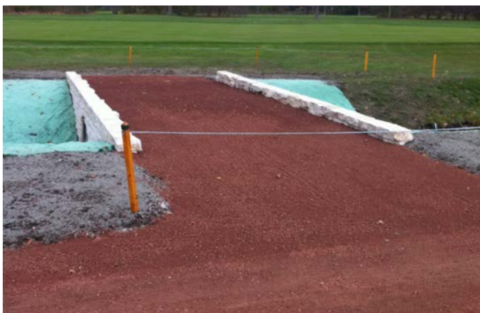
After each bridge complete and backfilled, staff finished off the grade with crushed red stone to match the existing path work at IHC.
