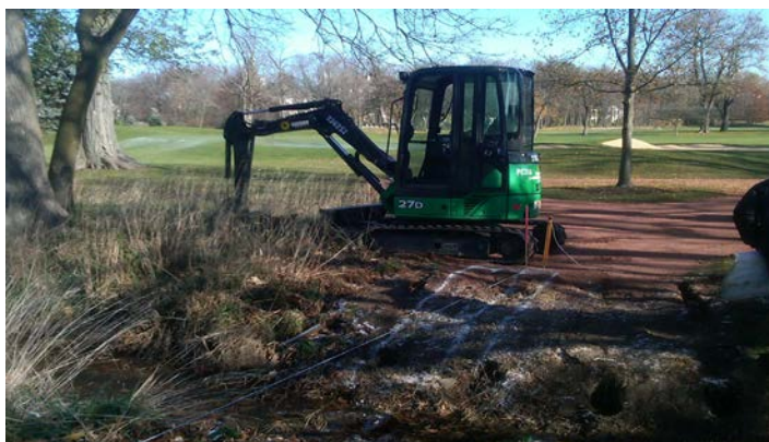
IHC rented a mini excavator to dig footers and properly place the pipes within the ditch.
