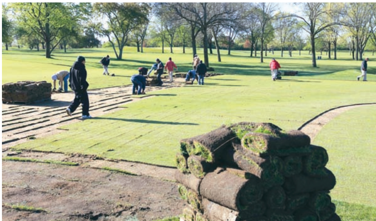
The clock starts ticking. The crew takes advantage of the dry spring to strip a low area in a fairway. The ground will be re-contoured to increase surface drainage and the sod replaced within a few days before the sod expires.
