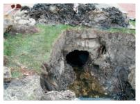
The hole was dug out and a new pipe was put in place.
