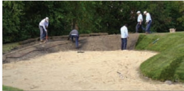
Installing drip irrigation while re-sodding the bunker face at the same time.
