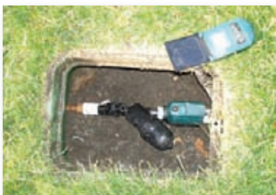
Tying the drip line into existing irrigation with control components was easy to do.
