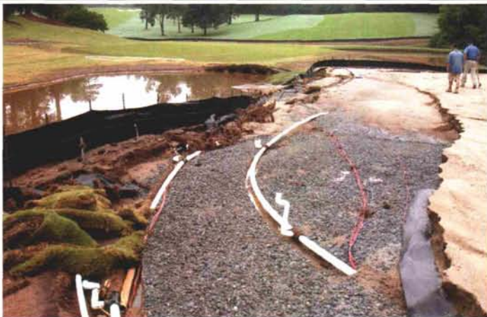
Covers can only do so much against a heavy rain on this green. This picture shows the uncontrollable aspects of a renovation that weather created – washing away and exposing irrigation pipes and gravel layers.
