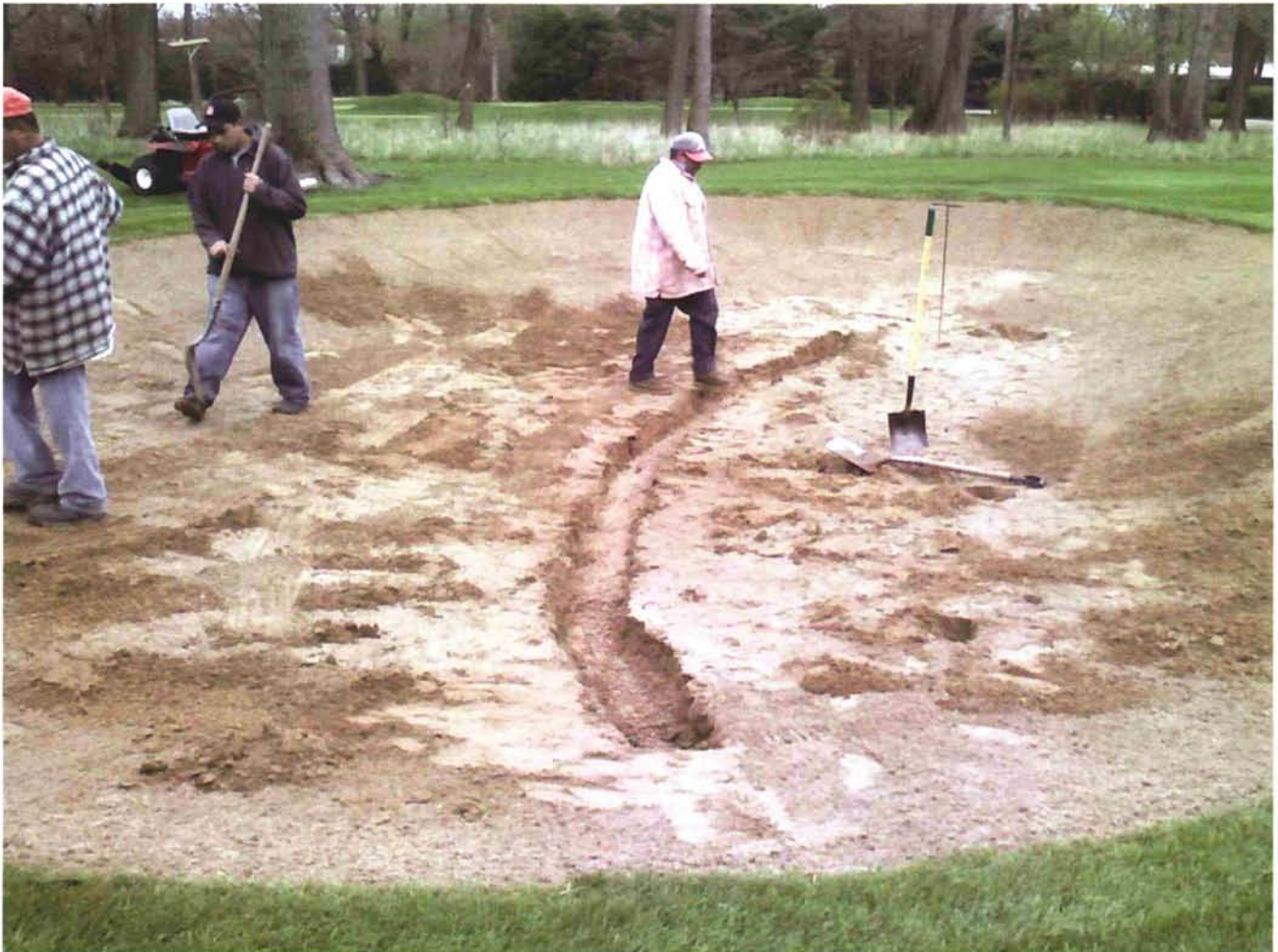
A few of the crew at Indian Hill remove old sand from atop drain lines in a bunker. New sand is used to backfill the trench, increasing the porosity to the tile line, thus increasing overall drainage of the bunker.
