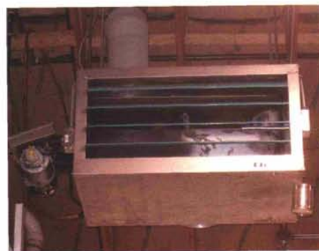
The new waste oil heater. Waste oil is pumped to the heater through the copper tubing to the left.
