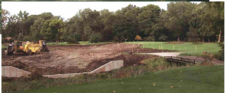
5th hole as construction begins and cottonwoods are absent. Pond excavation and weir structure are underway.
