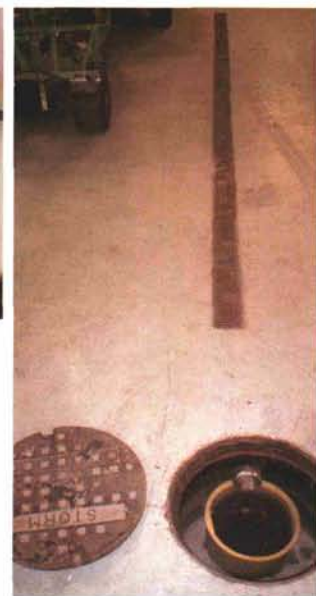
Catch-basin in floor with filter screen. The whole floor drains to a 20-foot trough that runs to the catch-basin.
