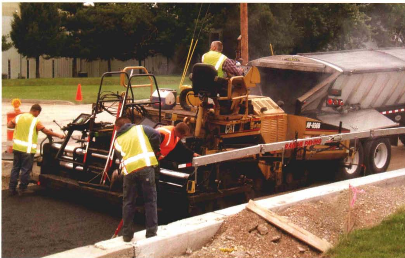
Caterpillar highway/road paver with laser-grade control system.
