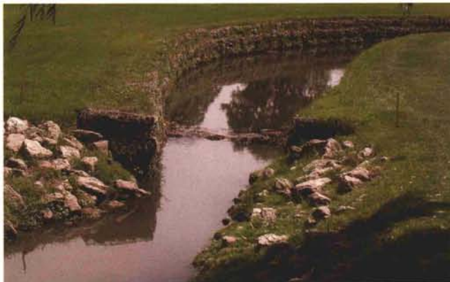
An example of erosion control for stream banks.
