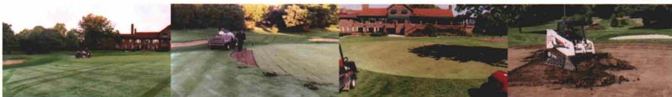
(L to R) Applying fertilizer and fungicide to existing green prior to removal of sod; removing sod from green; the green sod laid down just as it came off the green directly behind green complex on the clubhouse lawn; excavator removing 4" topdressing layer.
