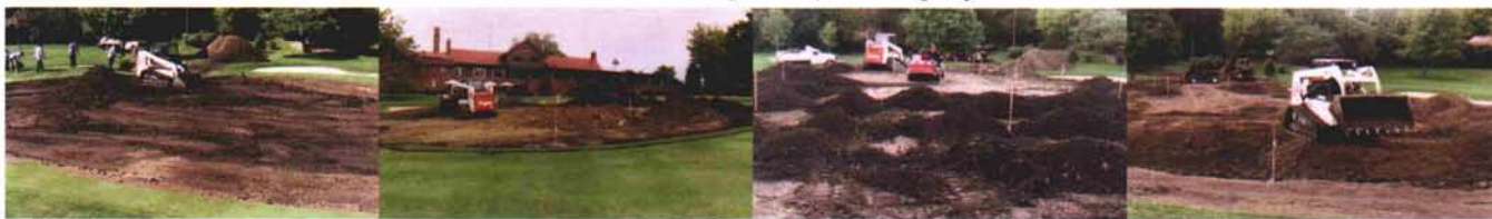
(L to R) Excavator removing 8" topsoil layer; excavator shaping green with fill brought in to reduce slope of green; hauling old topsoil mix back into green after fill had been added to reduce slope; hauling in old topdressing mix to go on top of old topsoil mix.
