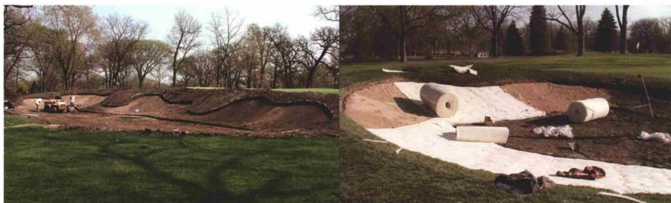
(Left) After old bunker sand was removed, as much as three feet-plus deep, the original bunker configuration became apparent. These contours were used as a guide to form the new bunkers as we built the edges by hand. (Right) Bunker construction in progress.
