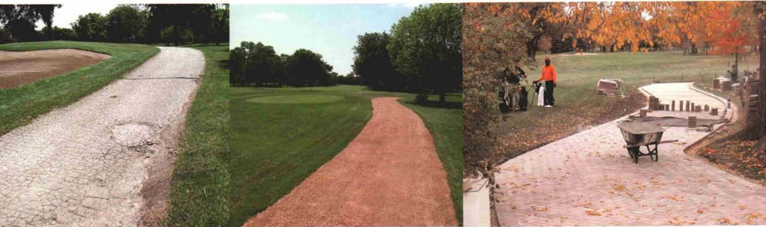
Renovation saw removal of all asphalt cart paths and replacement with stone paths in most cases. Where traffic is too heavy for granite gravel paths, rustic paving brick was installed, as on no. 10.
