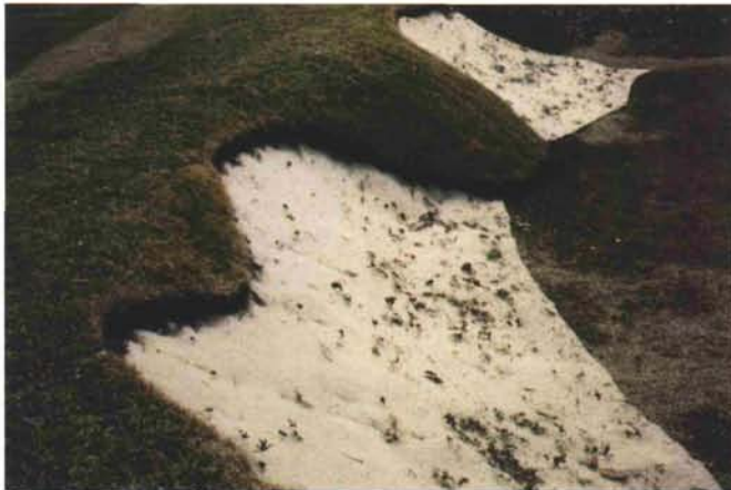
Sand Trapper bunker matting was installed along all bunker faces during construction.
