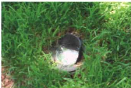
This is a fixed ground light. It would be used to light trees, shrubs, etc.
