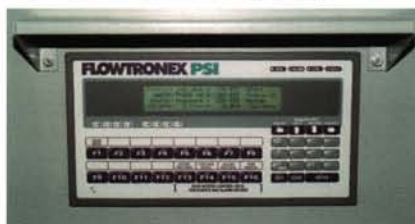
Data control pad for pump station.
