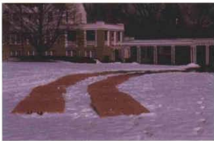
Plywood path for cement trucks to traverse to minimize golf course damage.
