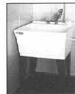
Wash tub with emergency eye-wash
