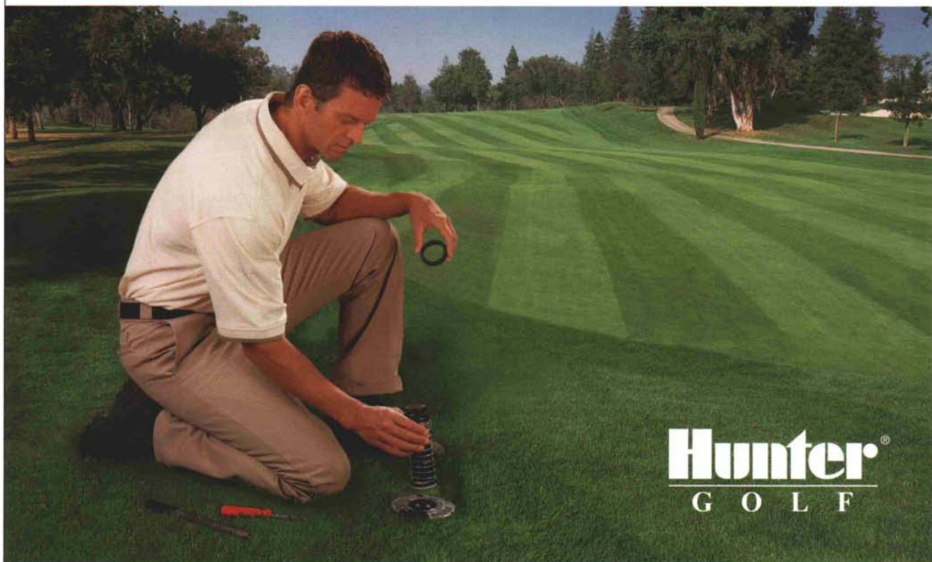
New Hunter RT replaces old Toro® riser in minutes and seats flush to flange.
