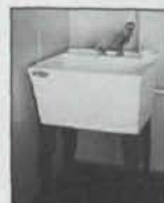
Wash tub with emergency eye-wash
