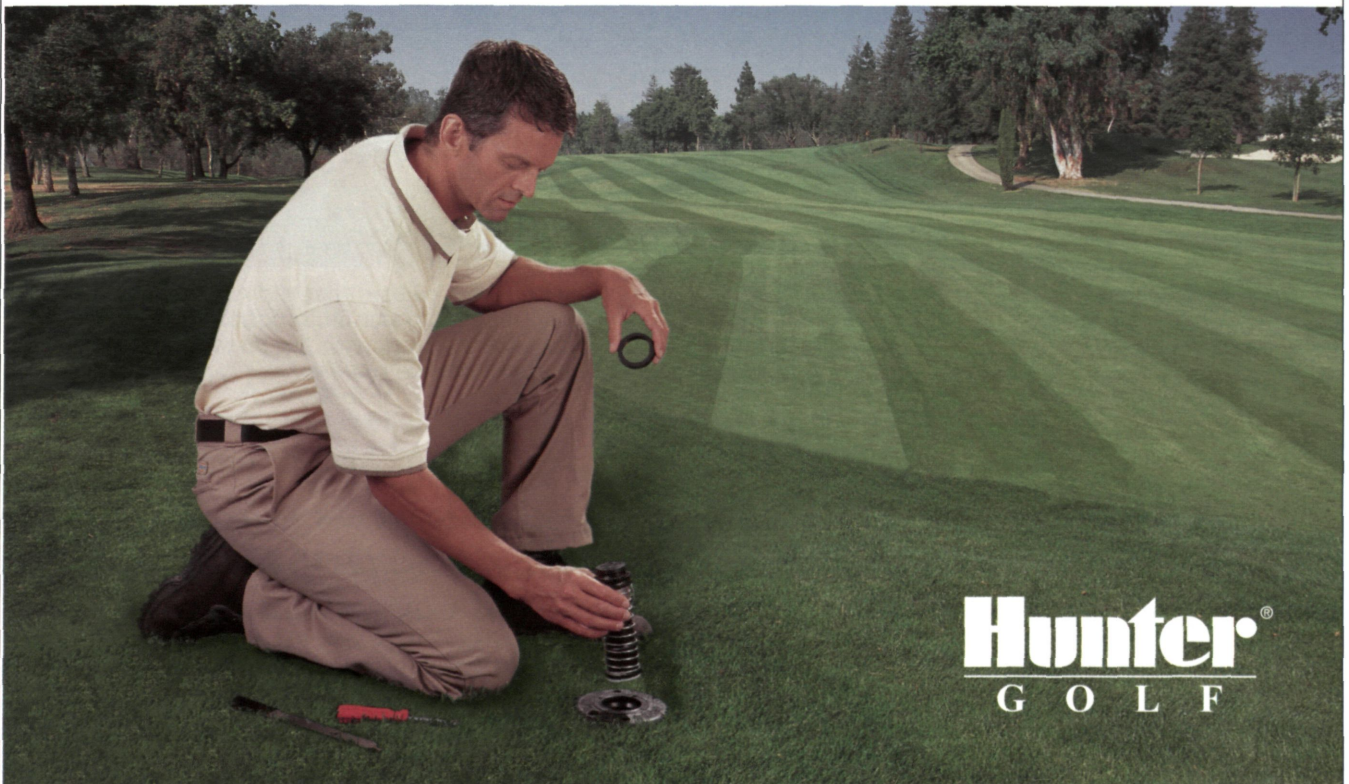
New Hunter RT replaces old Toro® riser in minutes and seats flush to flange.
