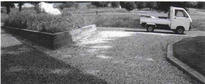
Sealing the service road to control dust.
