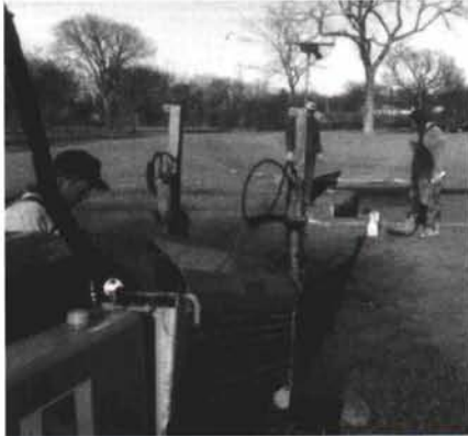
To eliminate surface disruption, drain lines can be put in with horizontal boring equipment.
