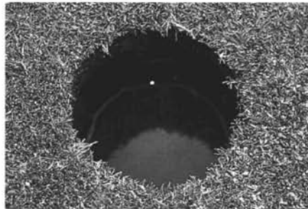
Standing water in the hole after a green has been deep-tine-aerified is a clear indication of poor subsurface drainage and the need to rebuild.
