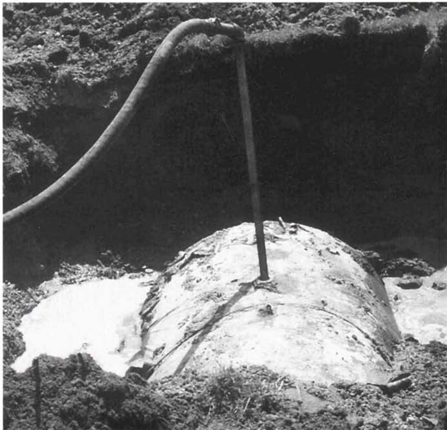
Pumping air into 3,000-gallon gas tank to get rid of fumes.
