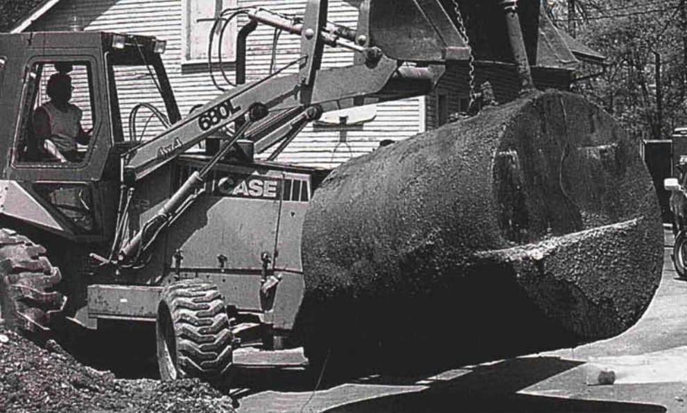
A 1,000-gallon heating oil tank.
