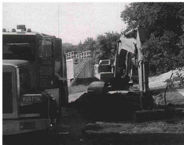
Redigging hole in cleanup of contamination. Portable water tank in background for excess water.
