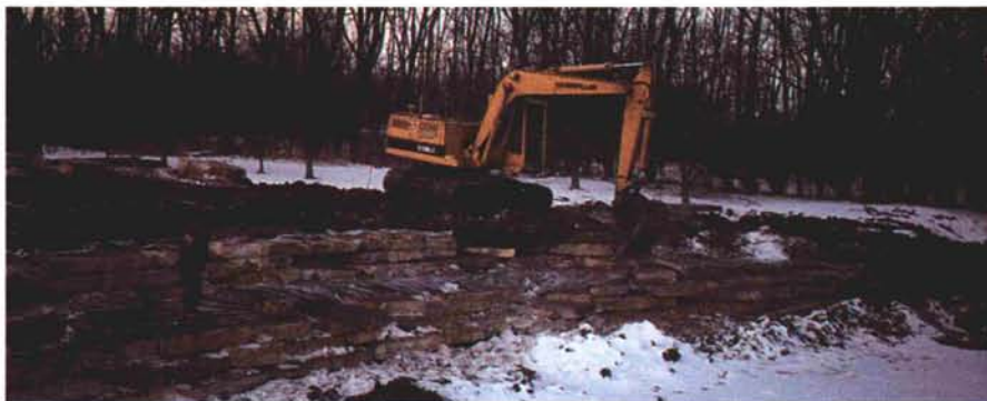
Construction on the 3rd hole pond.
