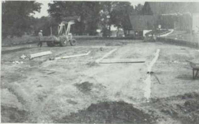
Rebuilding Practice Green at Butler National Golf Club.
