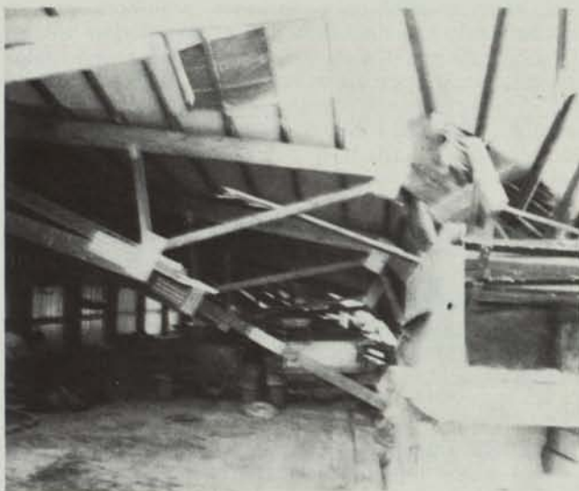
The heavy snow was too much for this roof at Ruth Lake C.C.
