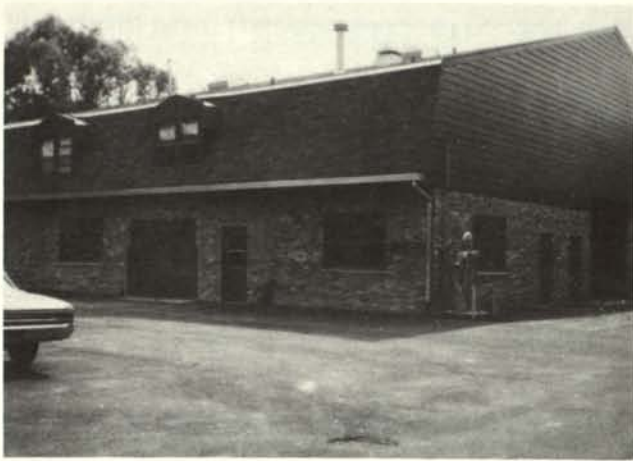
Maintenance Building at Sunset Ridge C.C., Northbrook, Illinois. 80' x 75'. Storage area 55' x 75'. Heated workshop, office and living quarters. Dom Grotti, Supt.
