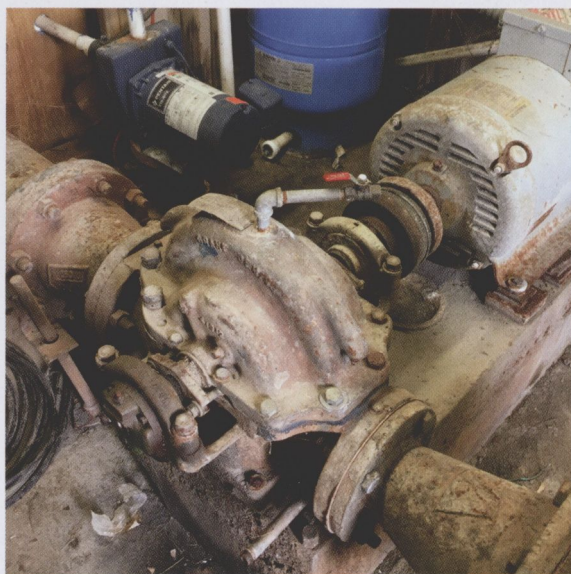
Centrifugal pumps are simple, rotated by a motor but need to be primed before they work.
