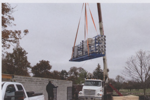
Like other components of pump stations, the r/o system was built offsite and set into place with a crane at Park Ridge CC.
