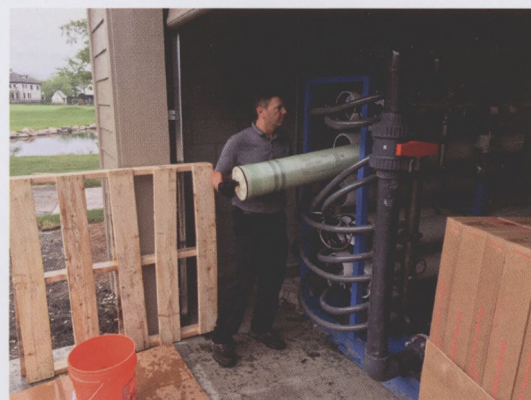
The long cylindrical tubes hold the filters (membranes) where the process happens.
