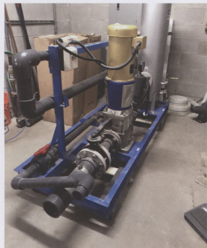
Pictured left is the 30 hp motor and booster pump that move water through the system. Notice that many of the fittings and components are corrosion resistant because once the water is cleaned, it is a bit caustic.
